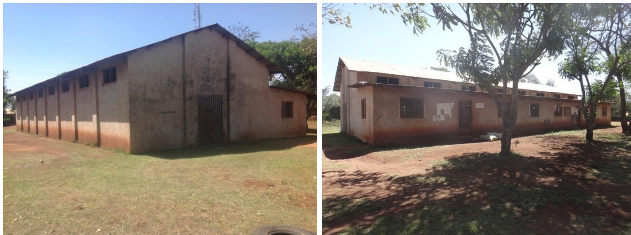
Plate 11: Rhotia Kati village warehouse in Karatu district
